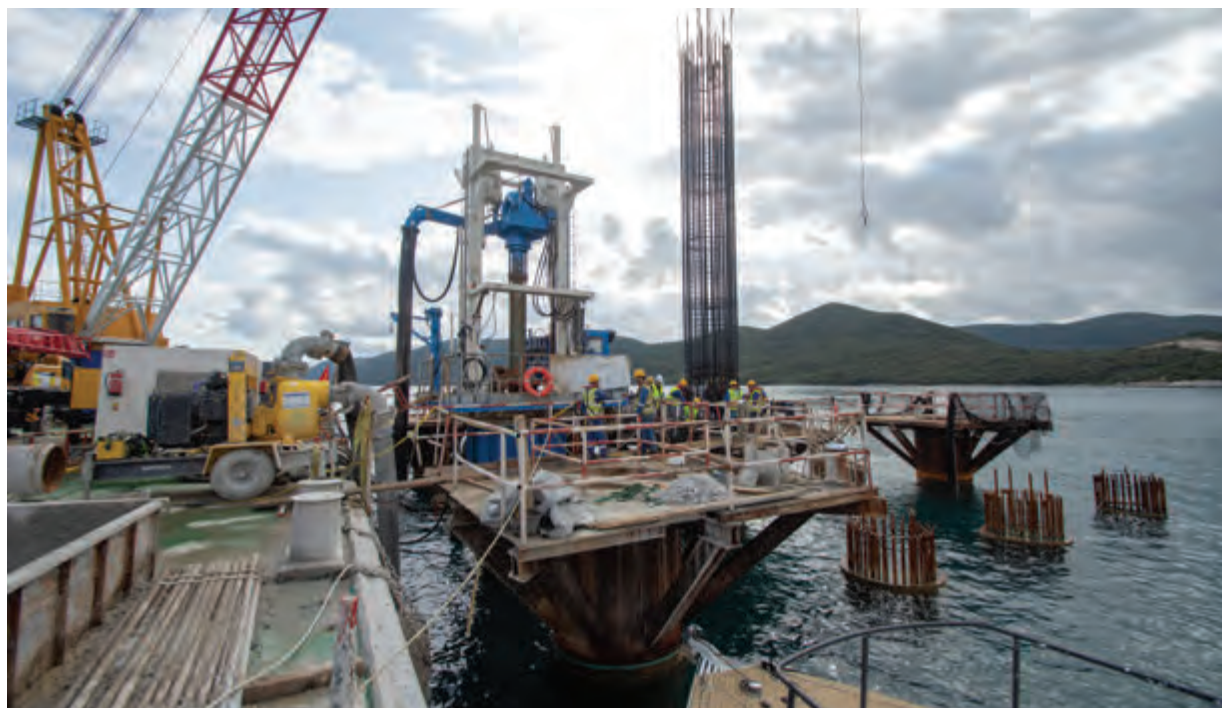
Piles of one pier site in different stages of making concrete filling: a drilling device is working on one pile, a reinforcing cage is being lowered into the adjacent pile, and several of them have already been prepared and concrete poured to the top, temporary constructions forming a working platform are in operation on the piles.
