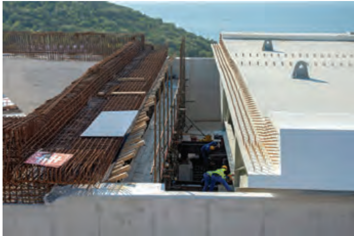
Completion of the span superstructure on abutment prior to the installation of transitional device.
