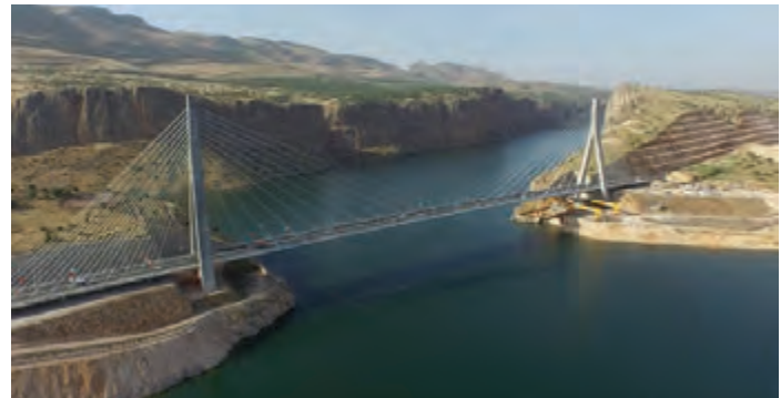
Cable-stayed bridge Nissibi across the Euphrates River in Turkey with a 400 m wide main span – this bridge and Črni Kal viaduct introduced Marjan Pipenbaher among the leading bridge designers in the world .
