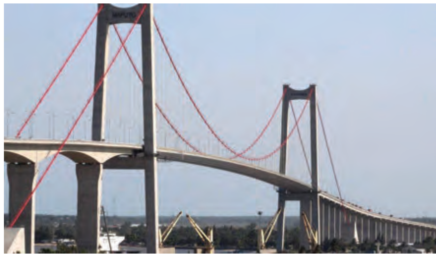
Bridge Maputo – Katembe in Mozambique, contractor CRBC
