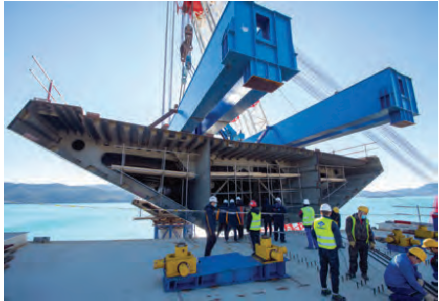
Lowering the segment of the steel girder to the installation location in the part of the assembly that is not suspended, the huge girders are used to temporarily support the structure, which weighs about 800 tons, during welding.
