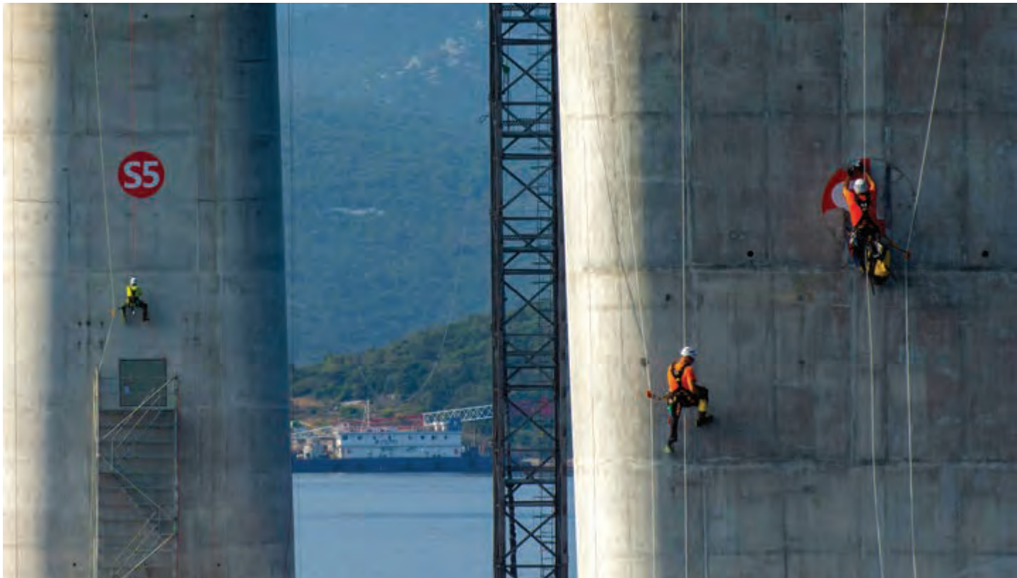
Cleaning the surface of newly completed piers and pylons is essential for the durability of the bridge, and the position of the workers indicates future challenges during inspections and maintenance.
