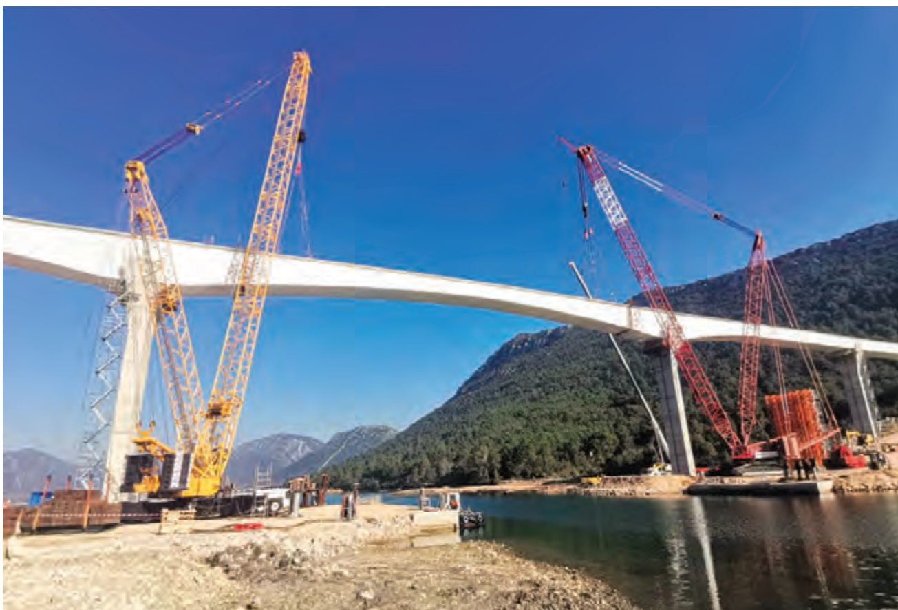
Construction site of the Ston Bridge, March 2022: erection of the central part of the structure over the bay
