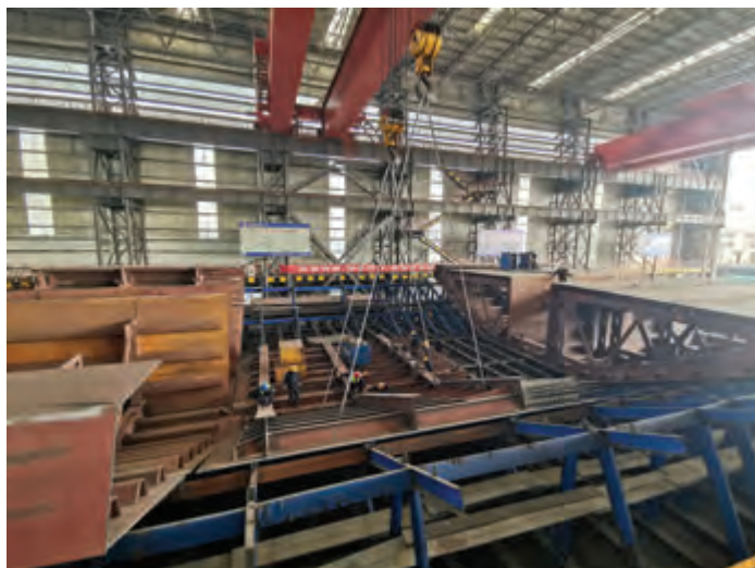
Production of steel elements of the Pelješac Bridge at a factory in China
