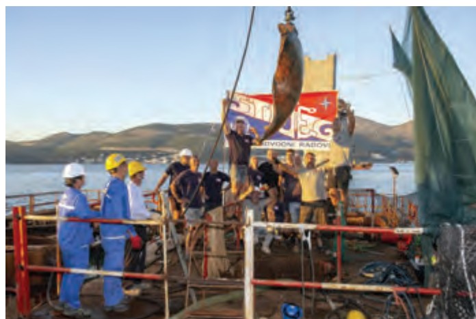
Removal of the deformed part of the pile pipe after underwater cutting
