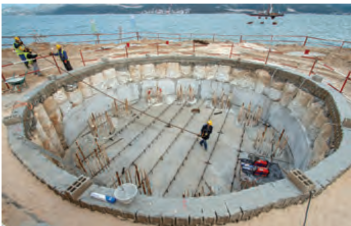
Construction of the pier S13 foundation, by the sea, on Pelješac: you can see the tops of the drilled piles on top of which the foundation slab was constructed.
