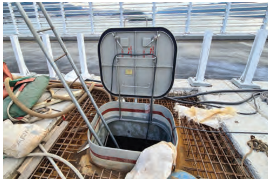
Entry into the bridge structure: door made such as those in ships, produced in the Radež shipyard, on the island of Korčula.
