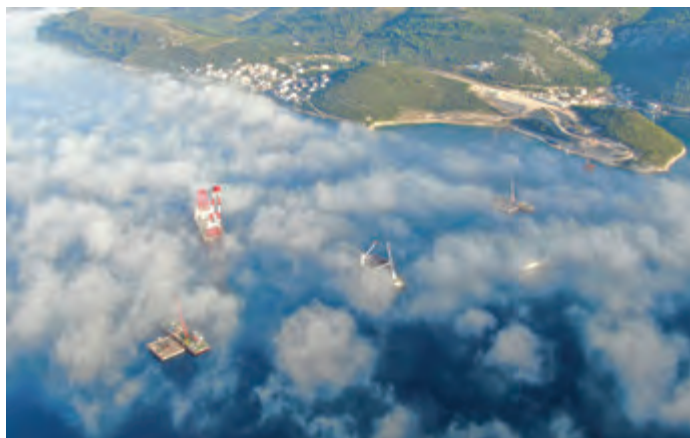
Construction site in October 2020.
