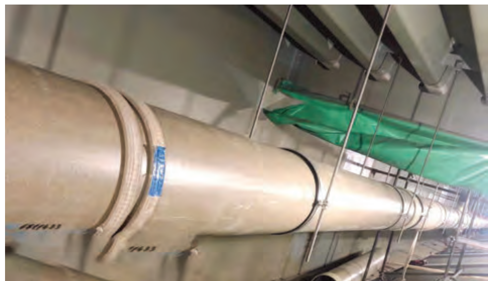
Drainage pipes from the carriageway inside the superstructure.
