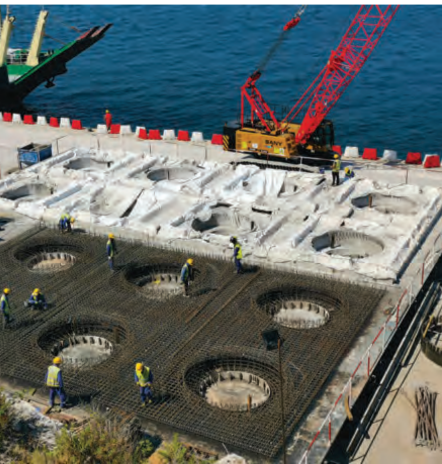
Casting concrete on parts of the bottom of the foundation slab (pile cap) on the operational coast near Brijesta, on the Pelješac peninsula.
