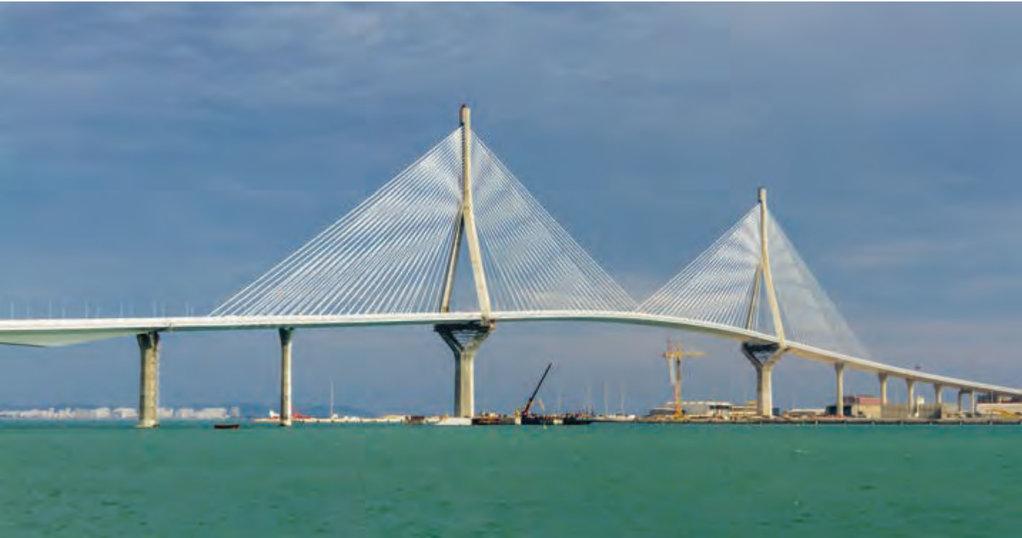
The Spanish Constitution of 1812 Bridge or La Pepa Bridge in Cadiz, with the largest span of 540 metres, completed in 2015.
