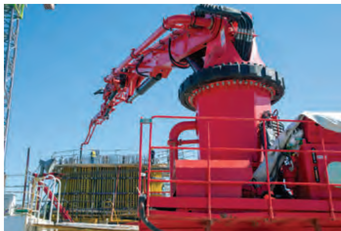
Pumping concrete from the ferry into the column formwork.
