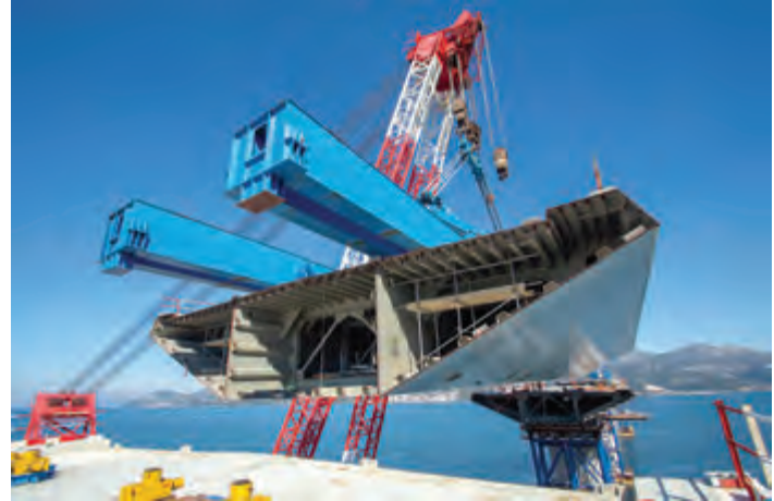
Connecting the first span above the sea, January 2021. |
