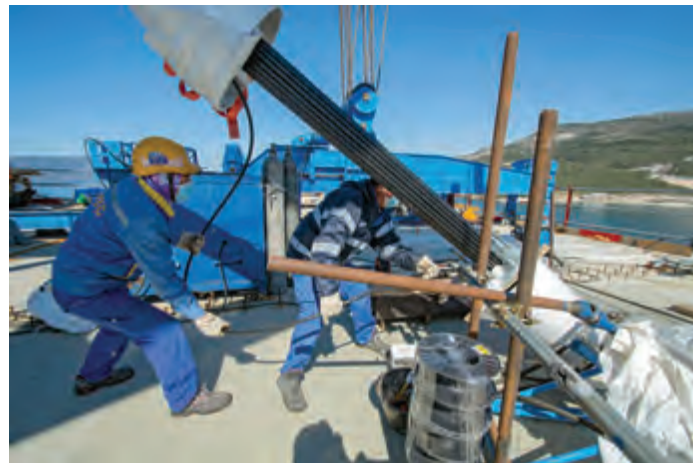
The inclined stay cables of the Pelješac Bridge consist of parallel strands, each strand holding 7 steel wires. The strands are pulled into the protective pipe on the construction site, then one by one the strands are tightened to a certain force. The stay cable consists of 55 to 109 strands tensioned with the same force.
