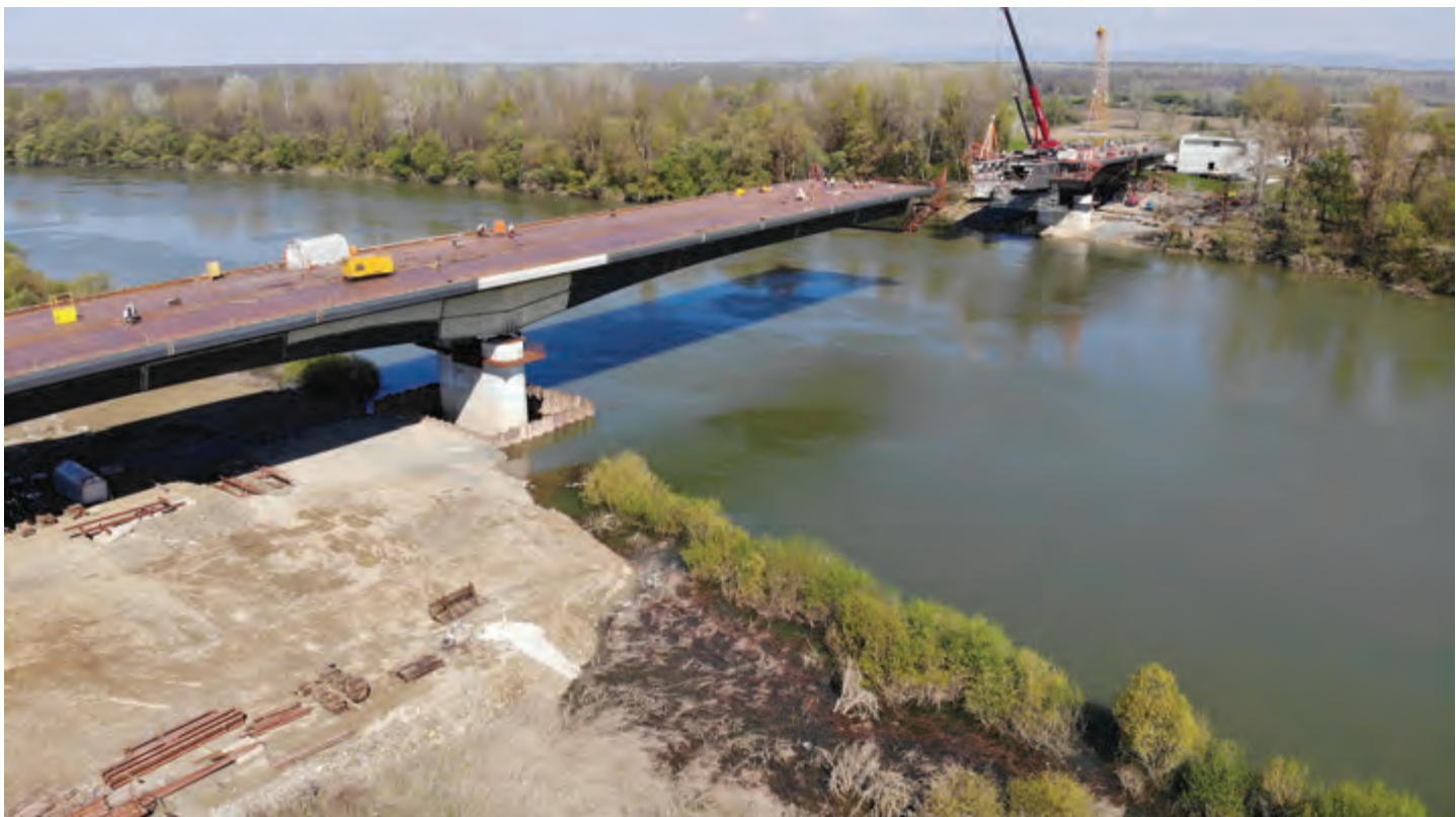
The Sava Bridge near Stara Gradiška, for the expressway, has a 462 m long and 23 m wide structure in which 4,650 tons of steel are installed.
