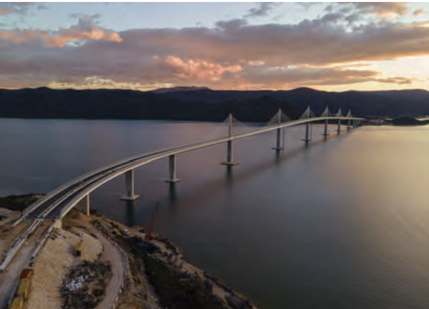
Final removal of defects, works are coming to an end. |
