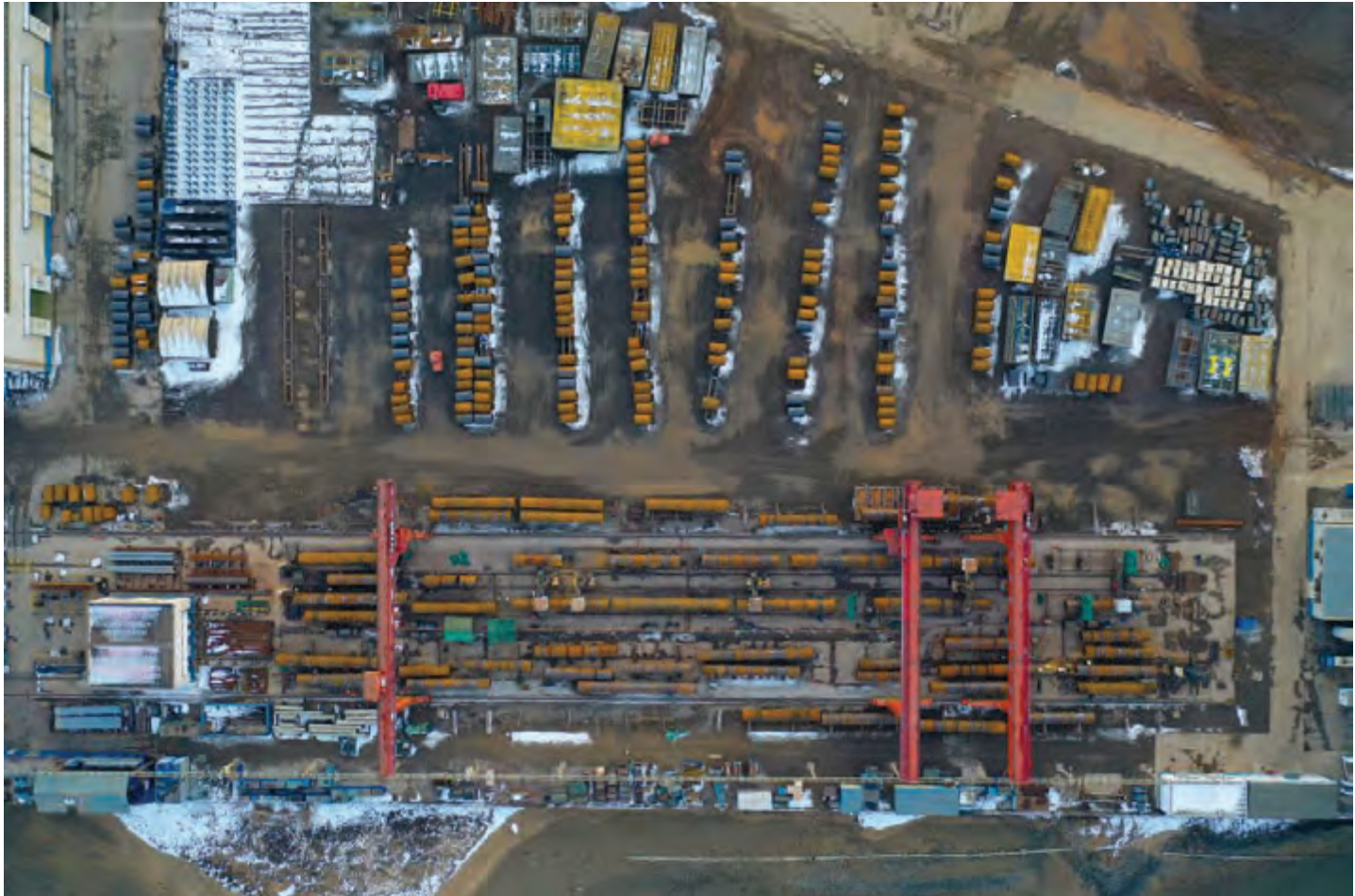
Forming piles in the factory: pipe pieces are welded together to the designed length.
