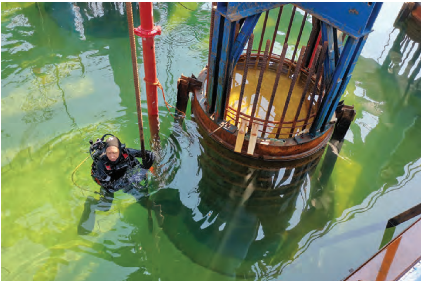
A very demanding part of the work related to the preparation of the pile caps was performed by divers (March 2020)
