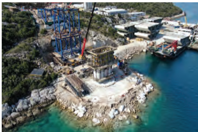
Execution of pier S13, March 2020, foundation on drilled piles made on a temporary embankment, scaffolding and formwork are moved by a crane, the concrete pump pipe at the bottom of the pier is visible.
