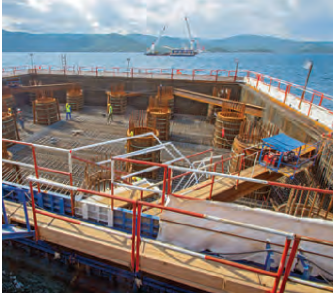
Interior of the box - formwork of the pile cap during reinforcement.
