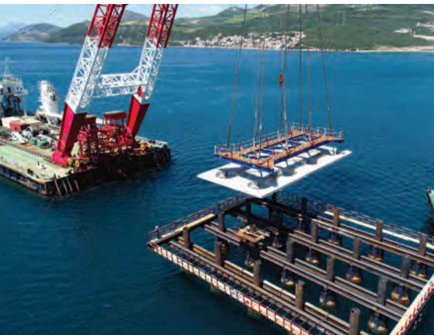
Transport and installation of one element of the bottom of the foundation slab (pile cap) on temporary supports in the pile extension: in the first stage, the pile cap formwork is formed above sea level. The auxiliary steel structure is later removed.
