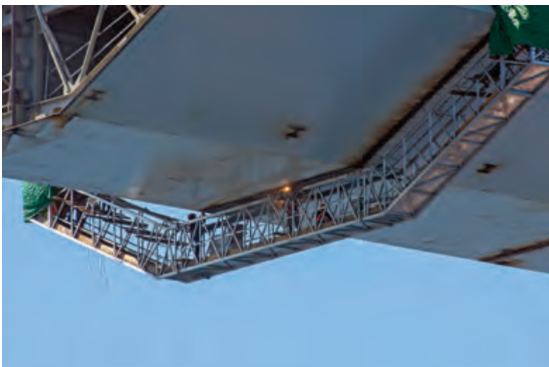
Welding of the circumferential joint of the bridge segments from below.
