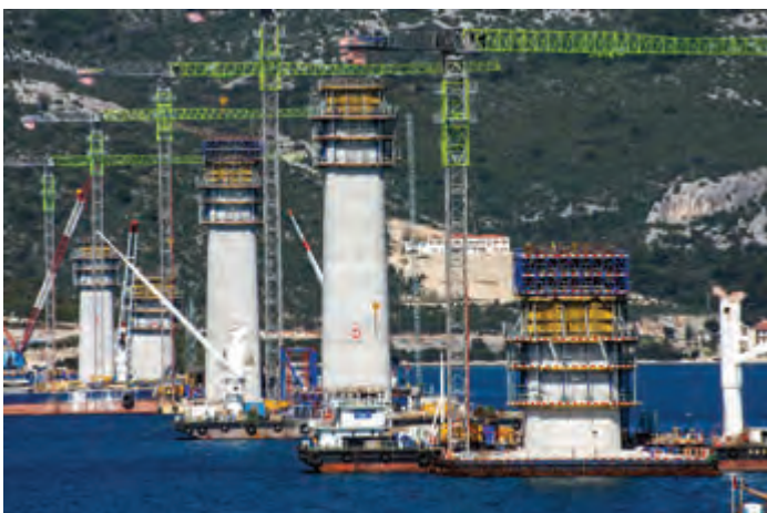
Construction of the lower parts of the pylon in 2020: each pillar in the sea is practically a separate construction site.
