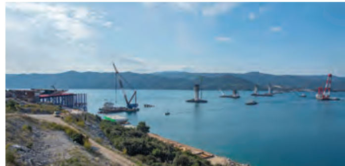
Construction site in March 2020.
