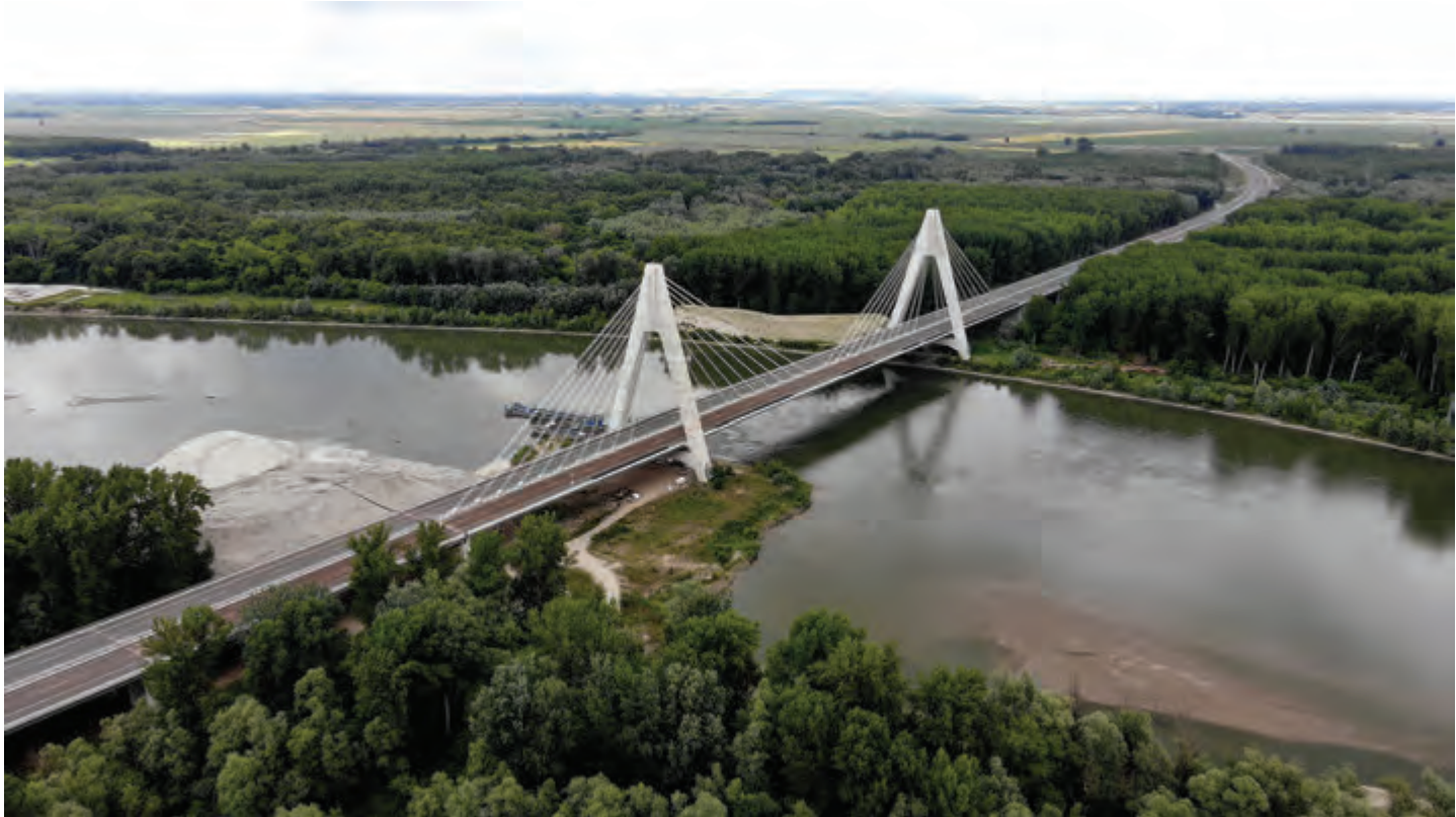
The Drava Bridge on the A5 motorway, Svilaj – Osijek – Beli Manastir, contains a 420 m long and 30 m wide composite structure in which 5,000 tons of steel are installed
