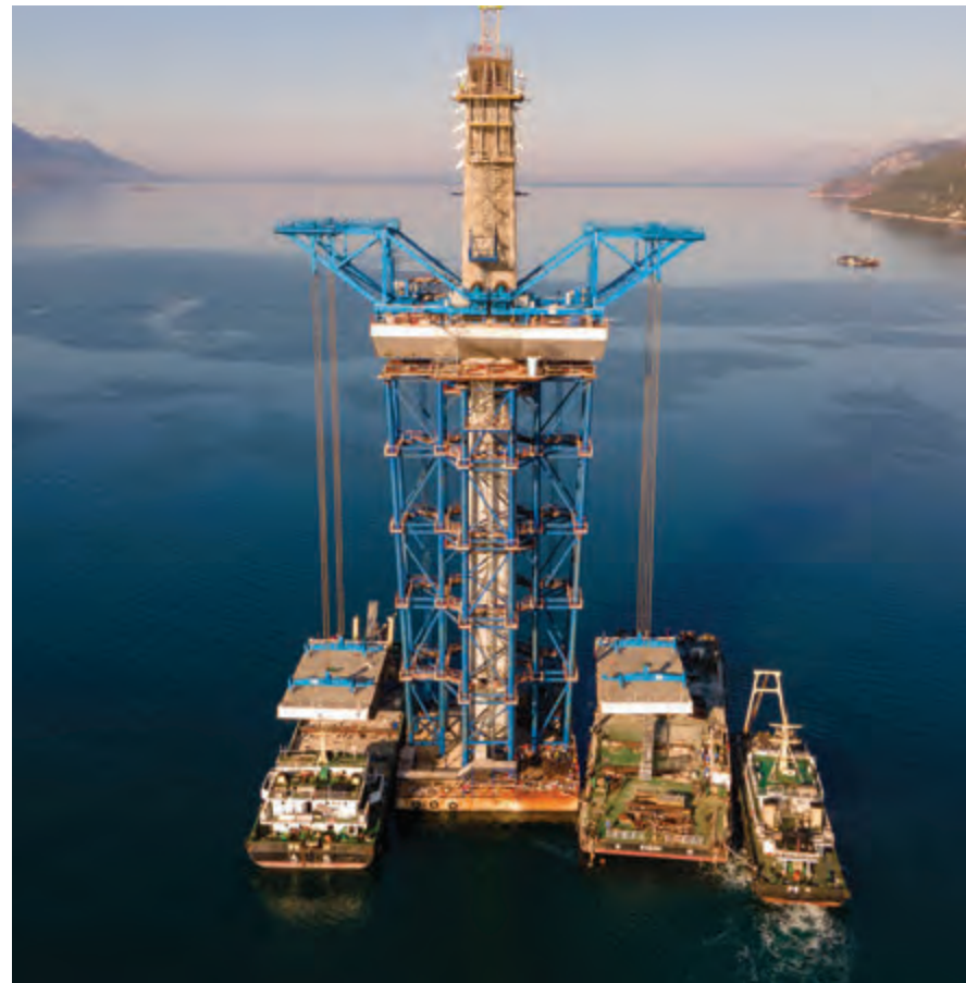
Lifting the first 12-meter long segments, which will be held in place by the stay cables, using derrick cranes on the base elements of pylon S7 in December 2020, the end parts of the steel saddles that will accept the stay cables are visible.
