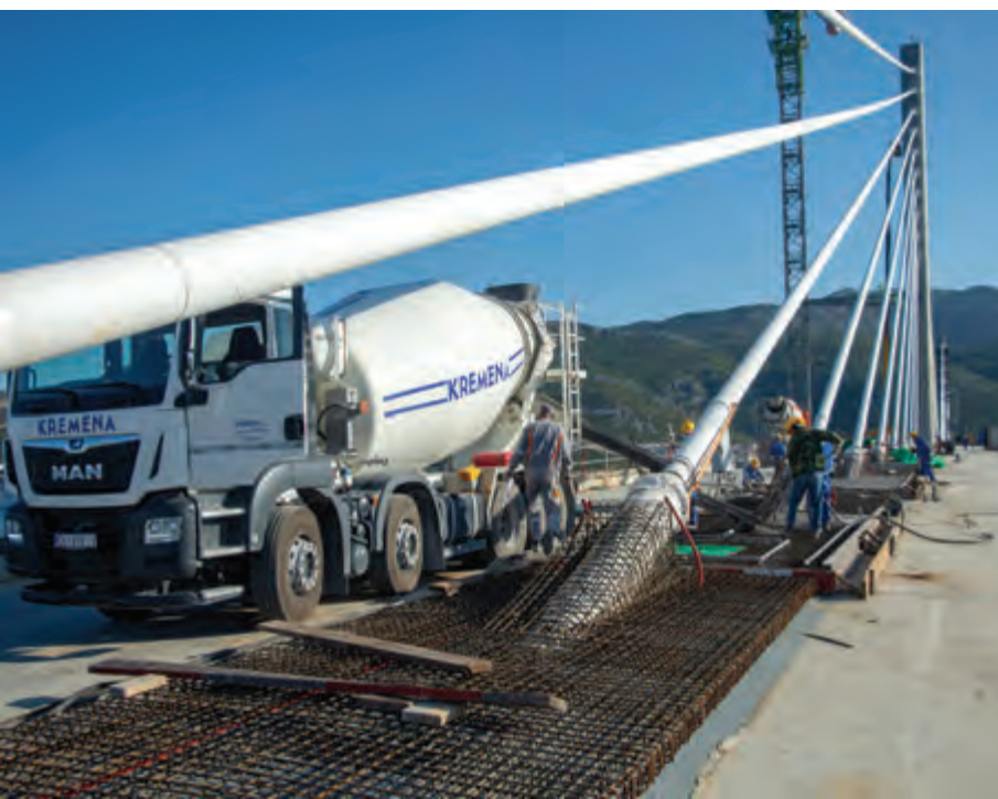
Concrete works on the central reservation on the bridge superstructure
