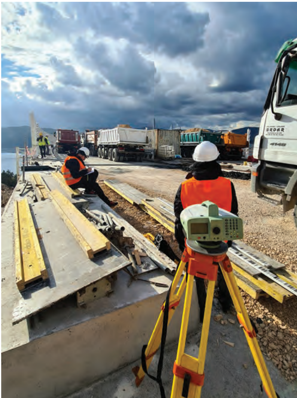
Geodetic equipment for monitoring displacements during load testing
