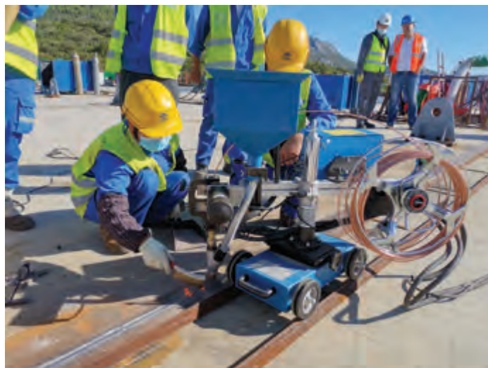
Semi-automatic welding devices were used to partially make the joints on the carriageway slab, the welds are filled, while most of the welds were made manually
