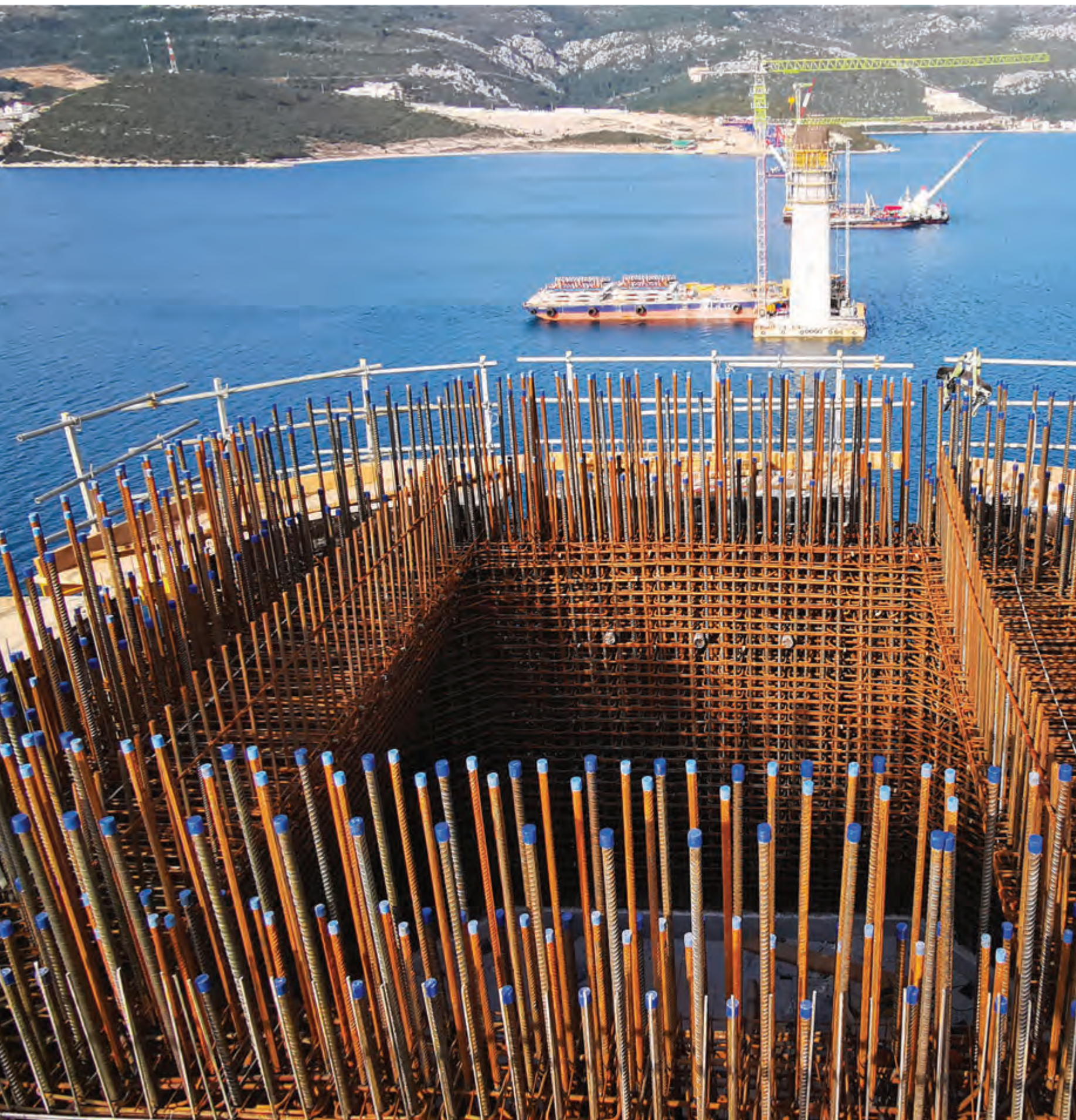
Reinforcement cage on the pier before concrete works
