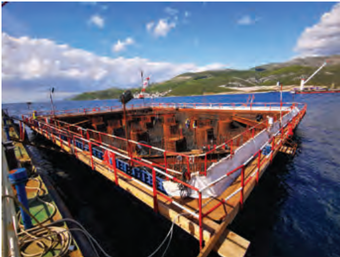
After the box above the piles is sealed and the sea is pumped out of it, the reinforcement of the pile cap is installed.
