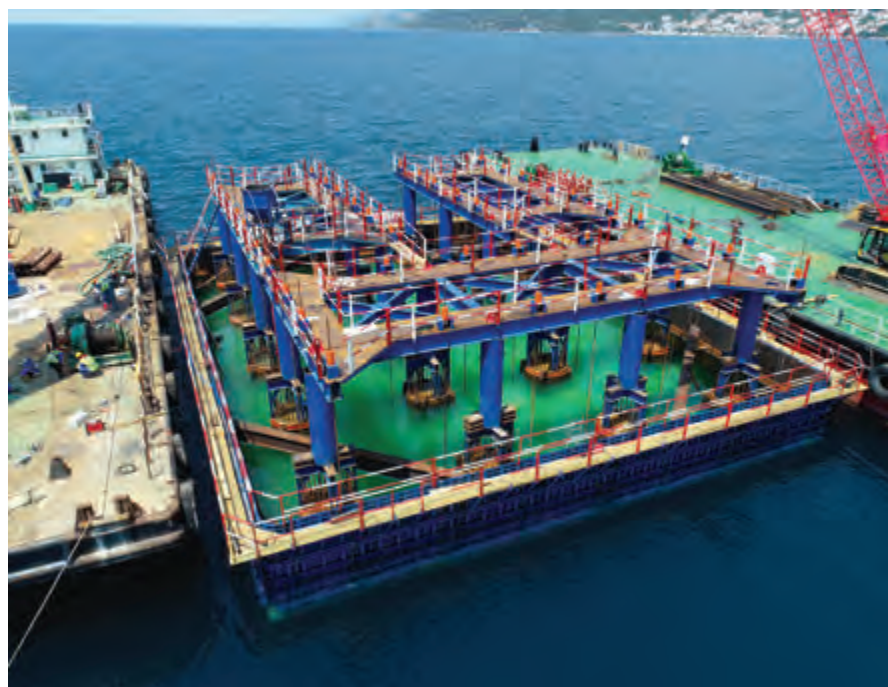
The formwork of the future pile cap is lowered to the designed height. Before pumping out the sea from the box, it is necessary to seal the openings around the pile tops (March 2020).
