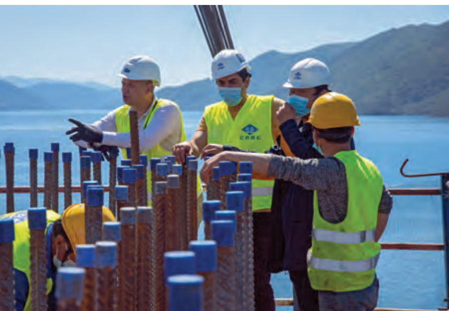
Supervision controlled and approved all works - before concreting part of the pylon (above) and before laying the reinforcement in the formwork of the main girder
