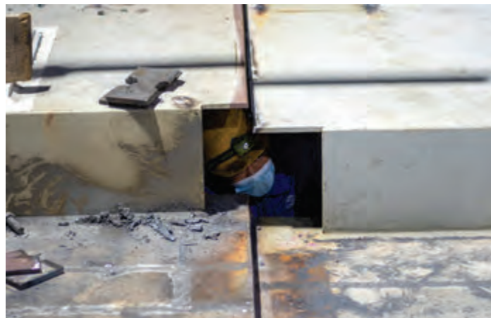
Fine-tuning of the position of the bridge segments before the final connection
