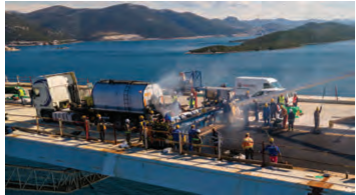
Installation of asphalt surface on the carriageway, October 2021. |
