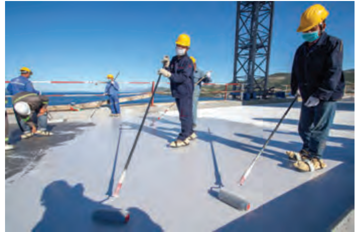
Laying of waterproofing on carriageway surface, October 2021
