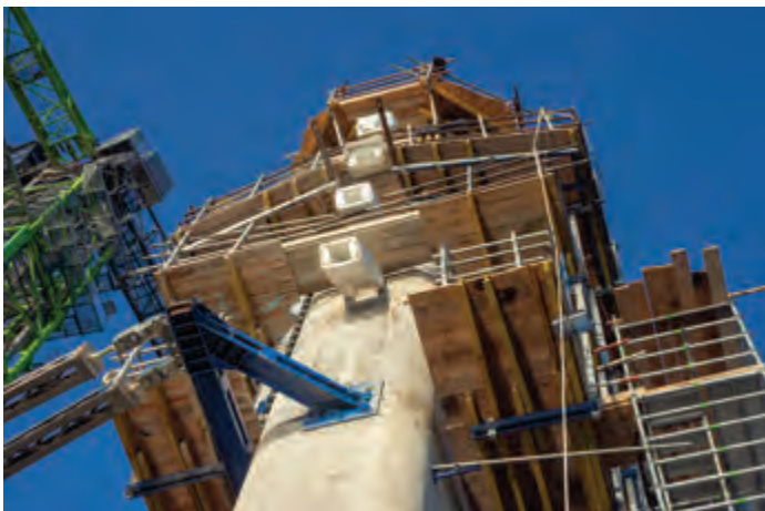
The full part of the pylon above the carriageway during construction - the saddles of the stay cables are prepared for fixing the steel strands.
