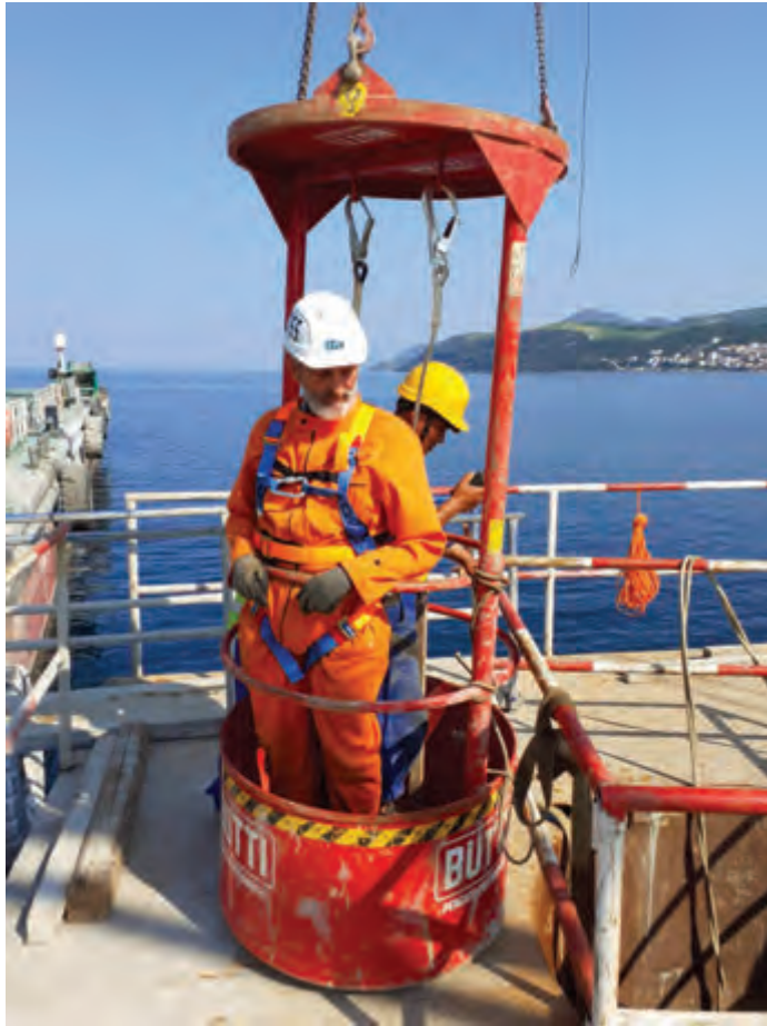
The basket for inspecting the interior of the pile is lowered by a crane into the cleaned part of the pipe, to the bottom of the space that will be filled with reinforced concrete. Our supervising engineer and a Chinese operator are in the basket.
