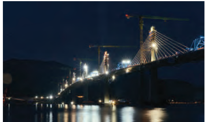
Lifting the last steel structure segment, July 28, 2021. |
