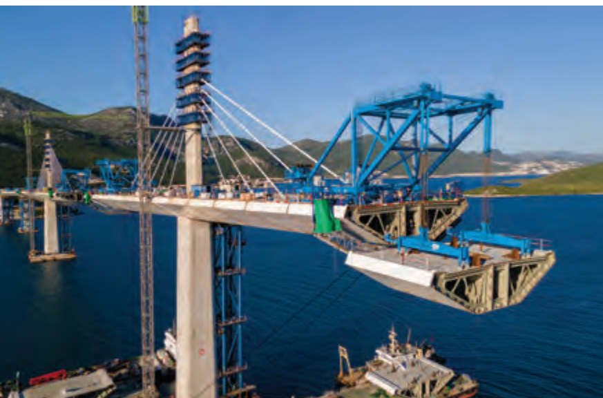
Pylon S6, balanced cantilever construction, May 2021.
