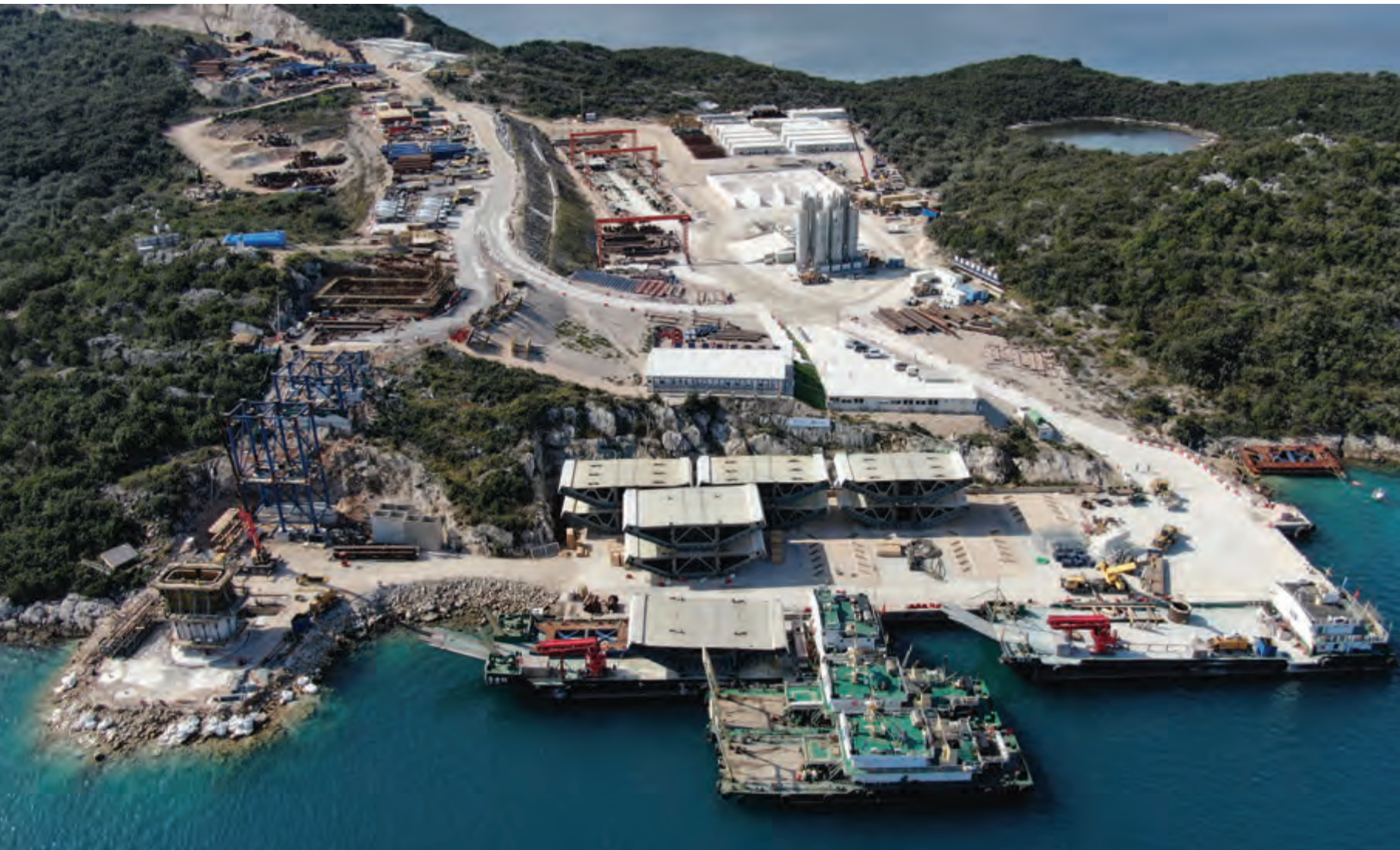
Construction site of the Pelješac Bridge in March 2020, tidy and well organized |
