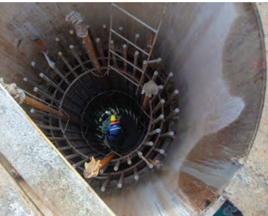
A view of the interior of the cleaned pile into which the reinforcement has been inserted. Old gloves protect the tip of the four pipes used to test the integrity of the piles after concrete was poured (Crosshole Sonic Logging)
