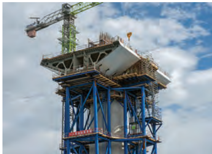
First steel elements on the scaffolding next to the S5 pylon – June 2020
