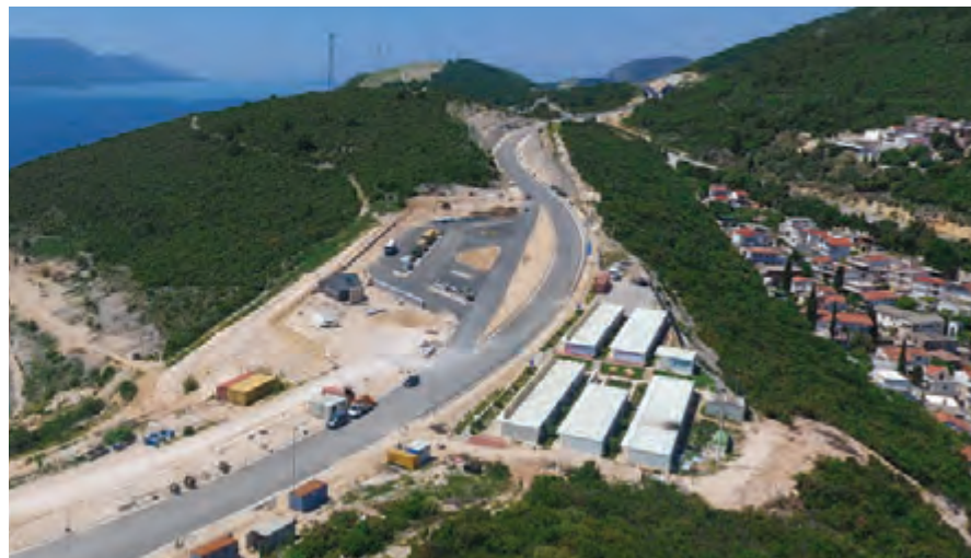
Access to the Pelješac Bridge from mainland – road service area Komarna under construction
