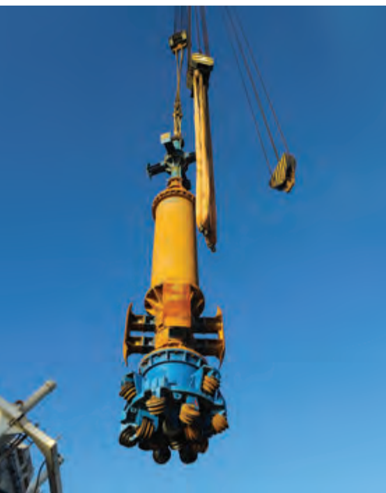
Drilling head for RCD drilling of the material left in the pile pipe after driving.
