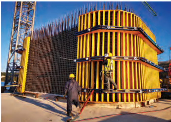
Formwork of the first block (section to be concreted at once) of the S5 pylon, December 2019, densely placed reinforcement indicated the use of self-compacting concrete.
