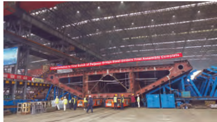
Production of steel elements of the girder span superstructure in a Chinese factory.
