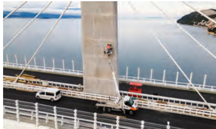
Installation of surveillance cameras on the bridge |
