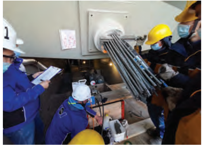
Tensioning of the inclined stay cable is performed using a compact hydraulic press, according to the given protocol, until the desired force is reached. Force is measured on the instrument in the centre of the image.
