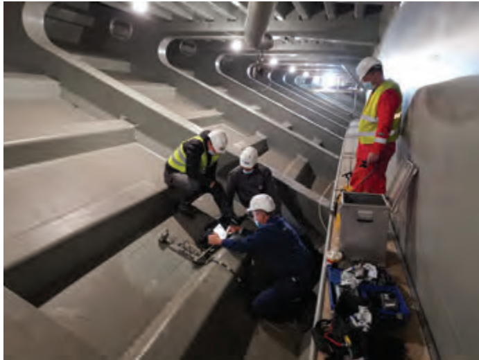
Inspection of welds with an ultrasonic device inside the bridge.
