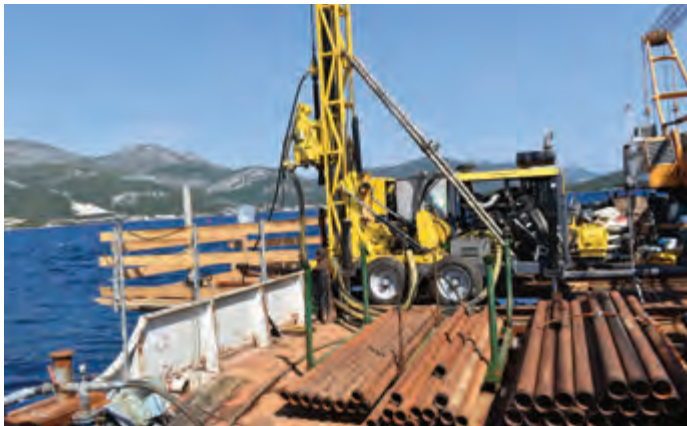
Geotechnical works at the bridge location: drilling of samples from the seabed is performed by pipes in which soil samples from a certain depth remain. Analysis of these samples determines the extent to which the soil is suitable for foundation.
