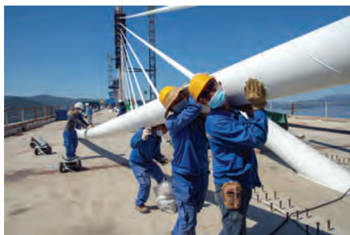
Installation of the protective tube of the stay cable, there are visible spiral protrusions that serve to prevent oscillations in special circumstances
