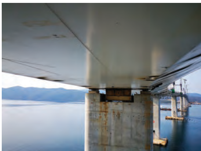
Bearings and rail at the top of pier S3 |
