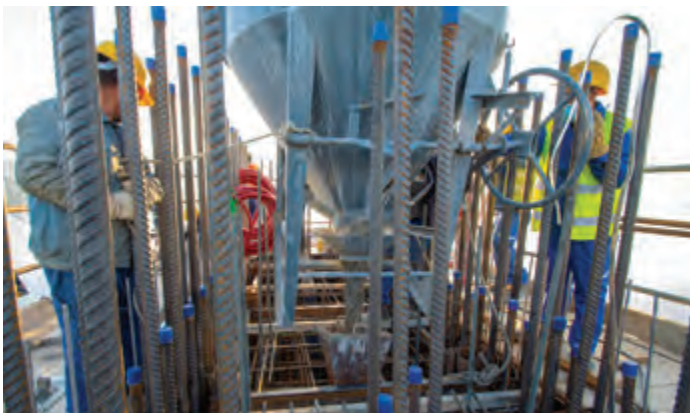
Concreting of the part of the pylon above the carriageway using a container - bucket that is lifted to the construction site by means of a tower crane. Dense reinforcement indicated the use of self-compacting concrete. According to the project, the highest concrete strength ever used for massive structure elements in Croatia was achieved.
