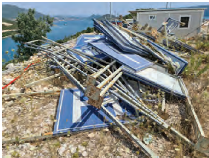
The stands of the boards with slogans are made of steel, and the foundations are concrete, but these unusual structures did not withstand the storm. If the wind knocked down a panel, a new one was installed immediately.
