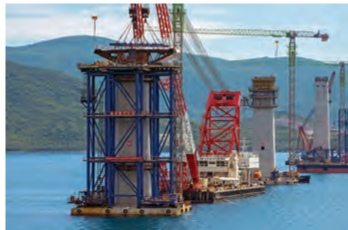
Installation of the first base segment in May 2020.
