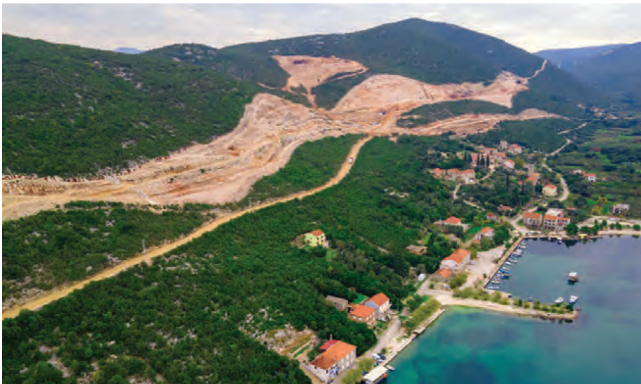
Construction site of the Brijesta junction on Pelješac, early 2022
