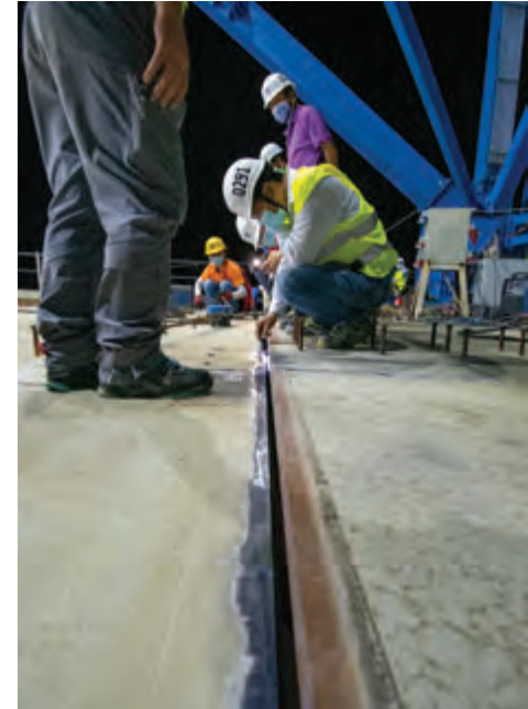
Fitting in the girder at night
