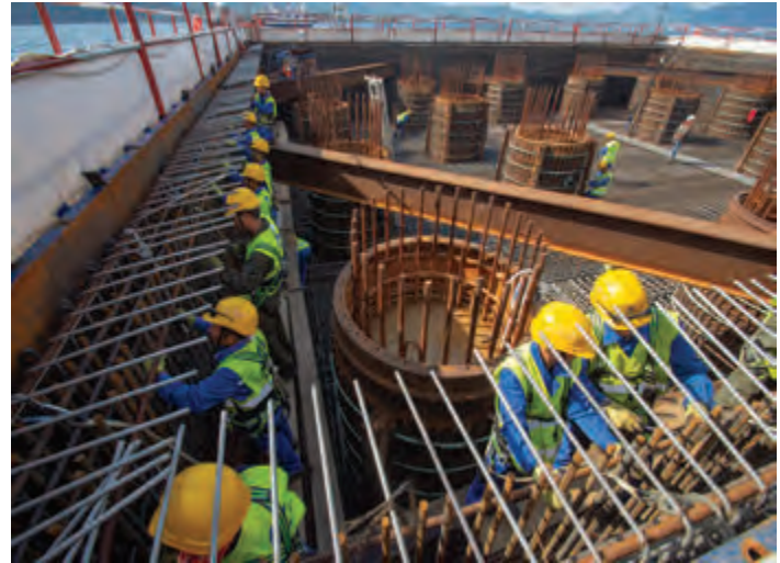
Chinese workers were very disciplined at the construction site, in the picture: reinforcing the pile cap
