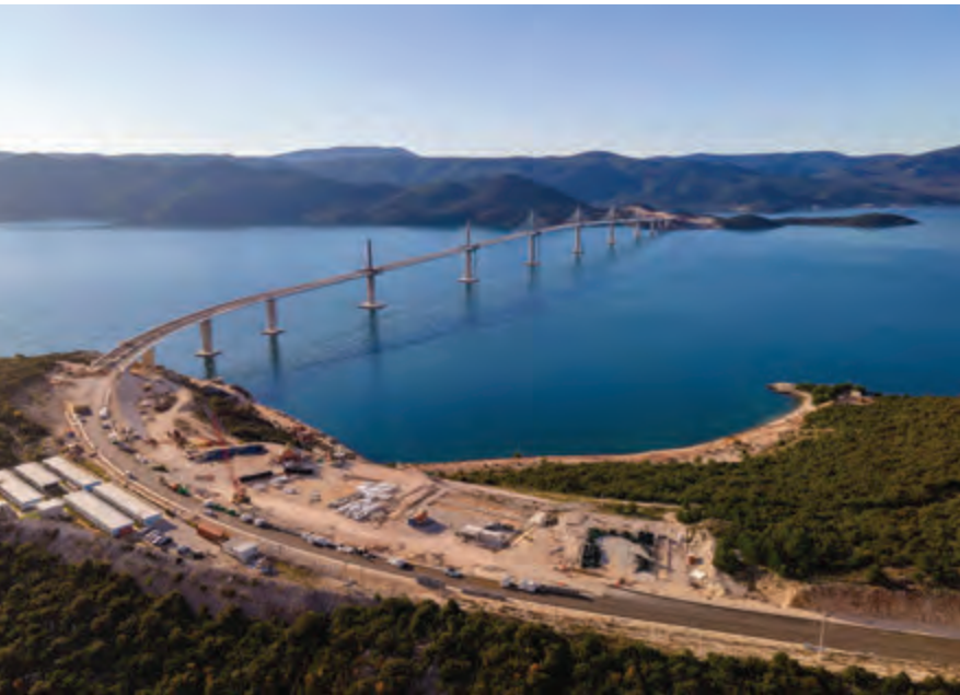
Final works in December 2021. |
