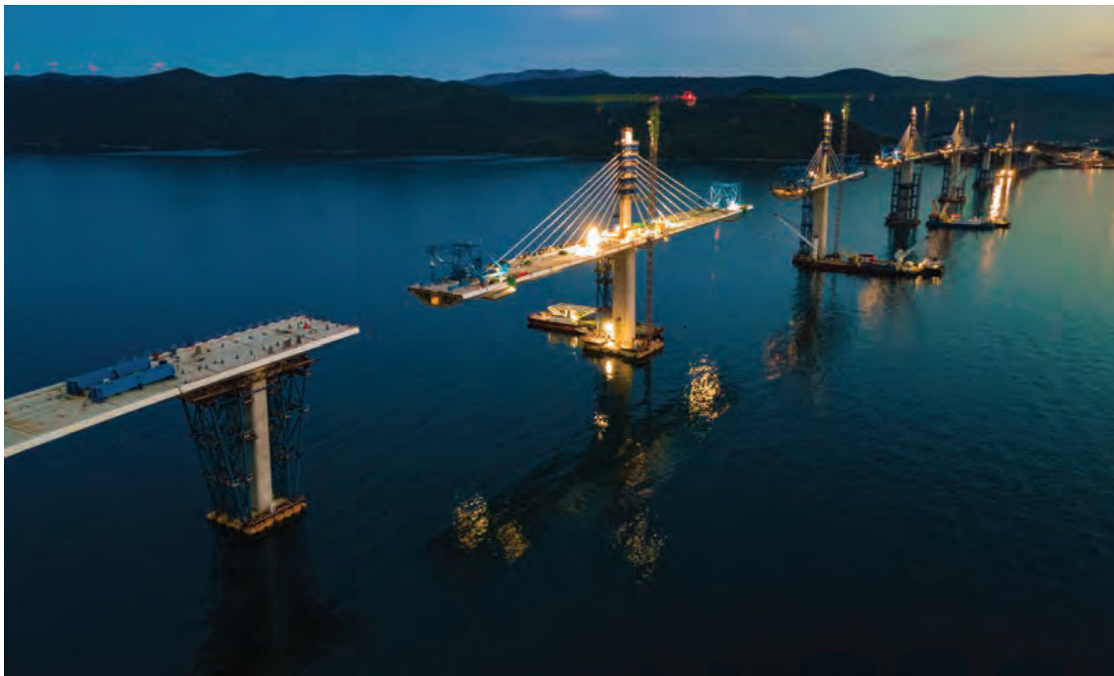
Pelješac Bridge in the Mali Ston Canal, cantilever construction with the installation of steel sections with the support of stay cables, May 2021 |
