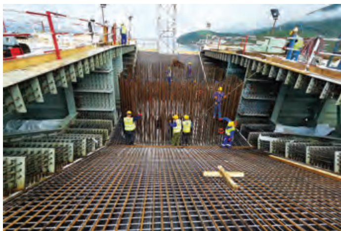
Construction of pylon S5, June 2020. The formwork and part of the reinforcement of the lower plate of the extended top of the pier were installed. Vertical reinforcement forms the outline of the future extension of the pylon above the carriageway. The dowels of the adjacent steel segments reveal the size of the space in which fixity of concrete and steel will be realized.
