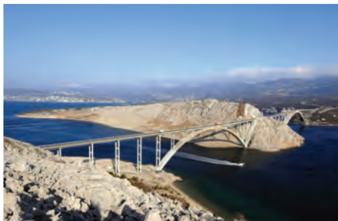
Krk Bridge, with reinforced concrete arch with the record span of 390 metres, completed in 1980.
