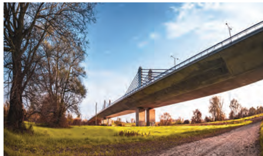
Homeland Bridge across the Sava River in Zagreb with a span of 12 metres, completed in 2006.
