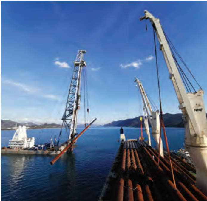
Driving the steel piles of the Pelješac Bridge: a ship with a hammer and a driving tower accepts the pile with a crane and turns it into the driving position.
