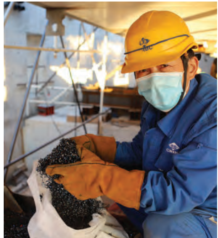
Chinese workers performing usual tasks at the Pelješac Bridge construction site.
