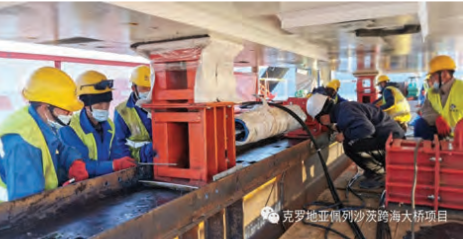
The segments above the land are pushed by presses to their final position in the structure - parts weighing around 180 tons gradually slide, pushed by hydraulic presses along lubricated channels on the scaffolding.
