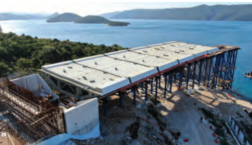
First segments of the Pelješac Bridge, on mainland, placed in their final position and prepared for welding - May 2020
