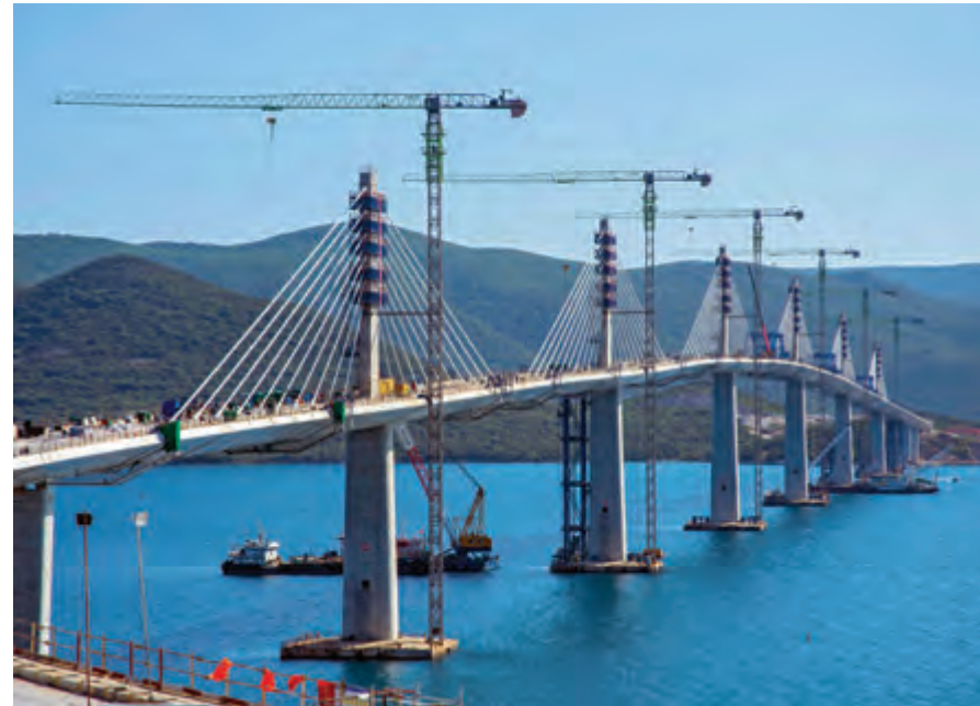
All six pylons in a row, from S5 to S10, August 2021.
