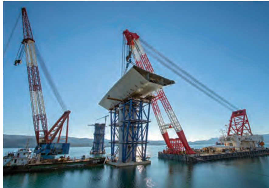
Installation of the girder segment on the S3 pier, October 2020
