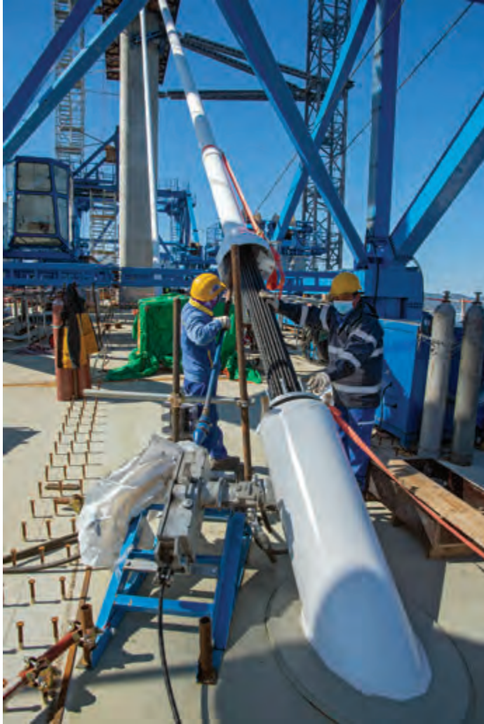
Pulling the rope into the protective tube from the carriageway – the strand of wires forms an inclined stay cable
