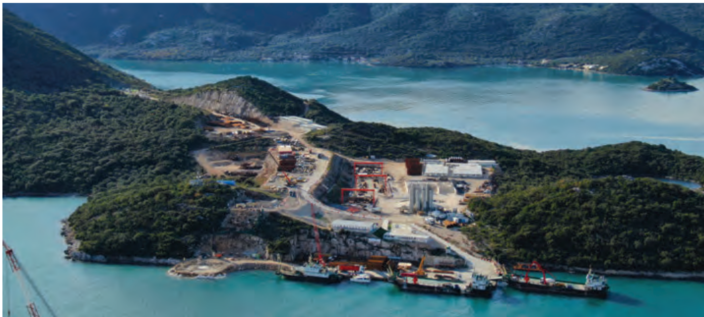
Construction site with facilities, site camp and operative shore near Brijesta on Pelješac at the end of 2019
