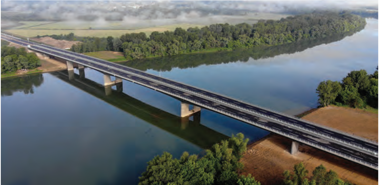
The bridge across the Sava River near Svilaj, on the A5 motorway, contains two parallel composite structure each 660 m long and 13.5 m wide, a total of 5,300 tons of steel installed.
