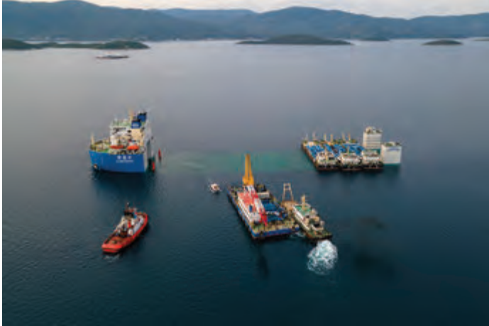
Demobilization of the construction site. |
