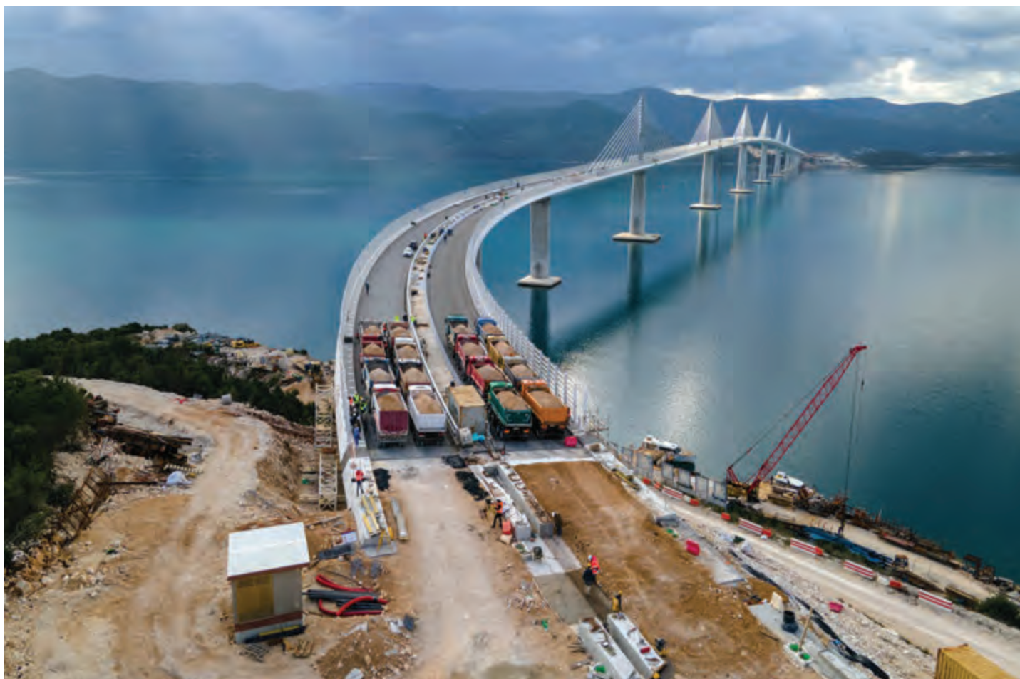
Load testing of the Pelješac Bridge by using twenty trucks of a weight of 40 tons each
