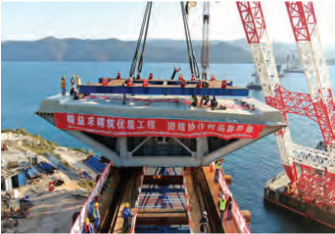
Lifting the first element of the steel structure on the mainland in March 2020. The segment was placed on the blocks by a floating crane, which, pushed by hydraulic presses, will slide together with the steel structure to its final position.
