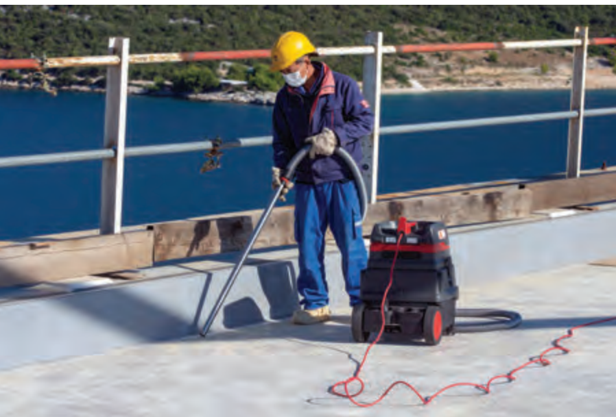
Cleaning of carriageway surface prior to laying one layer of waterproofing.
