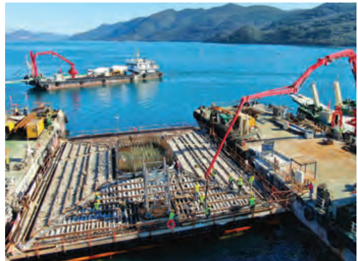
Concrete casting of the pile caps in the final stage - the upper formwork has been installed. The pile caps are probably the most massive concrete elements ever produced in Croatia, 3,000 cubic meters of concrete were installed in the largest pile caps.
