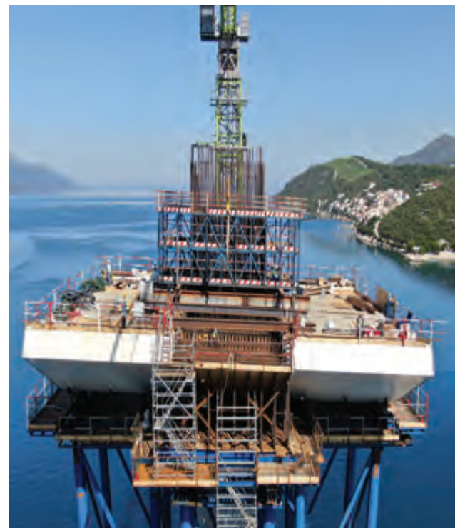
Connecting the first sections of the steel bridge structure with the pylon structure - formation of a rigid connection is additionally achieved by using prestressed cables. Construction of S5 pylon in June 2020: first steel sections along the pillar are put in place, on the scaffolding, between them, directly above the pier, concrete is being prepared.
